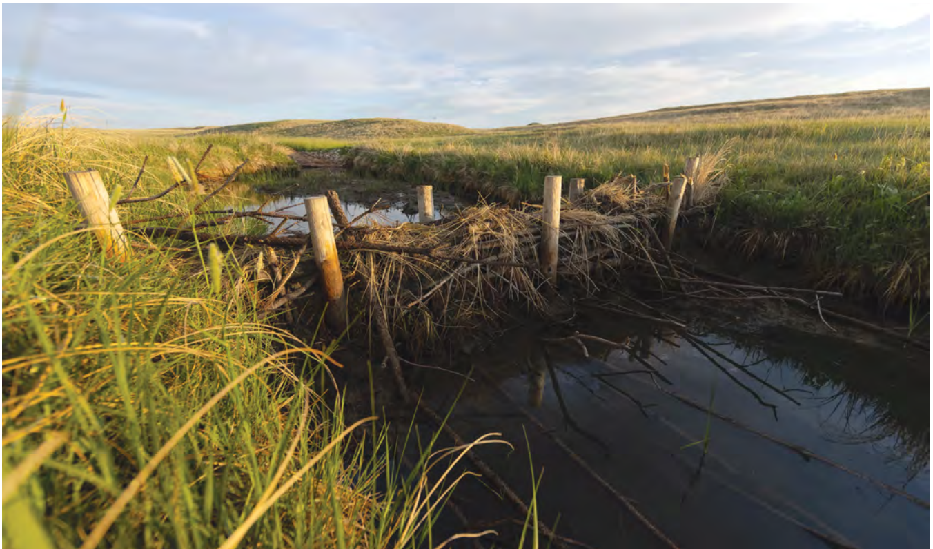
Figure 96: Beaver dam analogues seek to mimic beaver activity to slow and hold water while also trapping sediment and rebuilding a stream bed from incision. These images show the same BDA from upstream or above the structure (top) and from downstream or below the structure (bottom). The BDA works to slow and hold water, trap sediment, and rebuild the stream bed. The lower photo demonstrates that nearly 18" of sediment and water above the dam were accumulated in just one season of use. Photos © Joe Dickie, Generation Photography, Inc.
