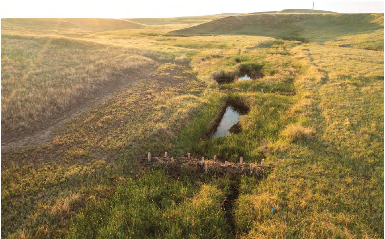
Figure 4. Beaver dam analogs work to slow and hold water in pools. Photos © Joe Dickie, Generation Photography, Inc.
