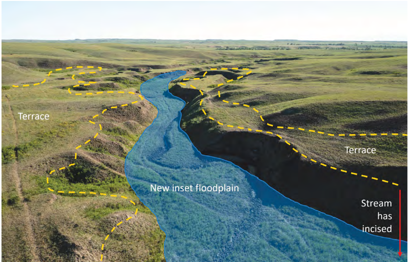
Figure 20: When a stream goes through an incision process, it no longer has easy access to historic floodplain areas, which become known as terraces. The inset stream now flows through a tighter channel with more erosive power. Photo © Joe Dickie, Generation Photography, Inc.
