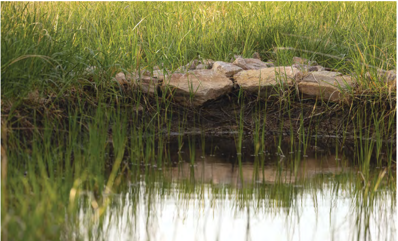
Figure 95: These photos show a rock Zeedyk structure used to prevent a headcut from advancing upstream. As shown in the lower photo, grass has already begun to grow through and revegetate the site, allowing the headcut to heal and preventing further erosion. Photos © Joe Dickie, Generation Photography, Inc.
