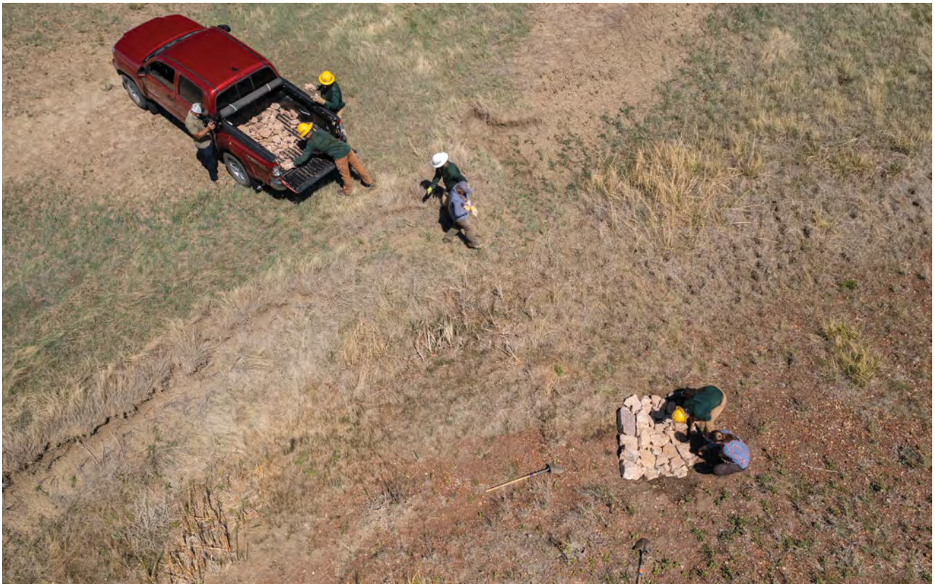
Figure 3. Boylan is working with organizations like The Nature Conservancy to install zeedyk rock structures in the stream beds to help slow down water, trap sediment, and reduce erosion. Photo © Joe Dickie, Generation Photography, Inc.
