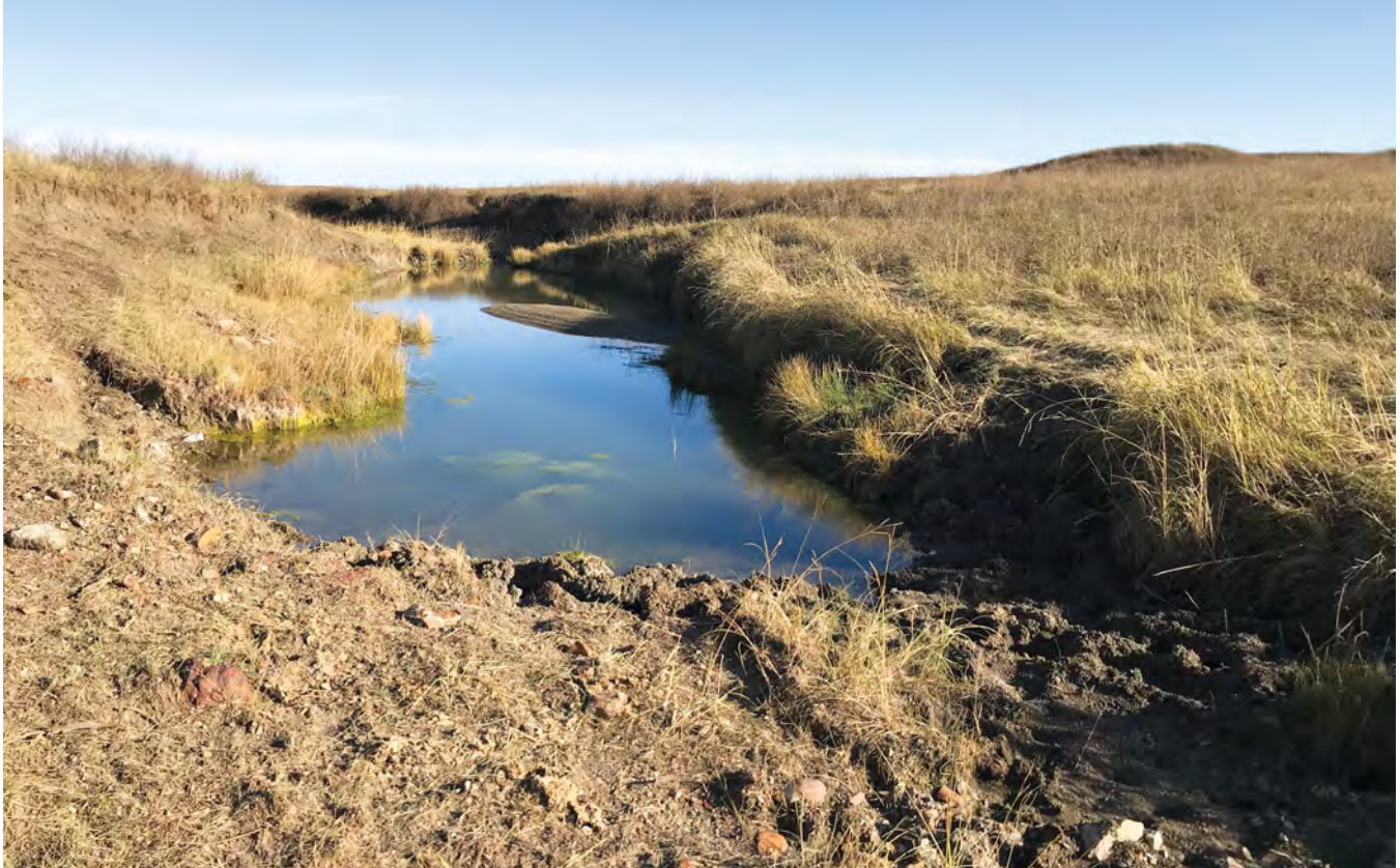
Figure 83: This channel has widened considerably in recent years due to streambank collapse, leading to shallower flow with little vegetative overhang to provide shade and habitat for aquatic life. Photo © Corissa Busse, TNC
