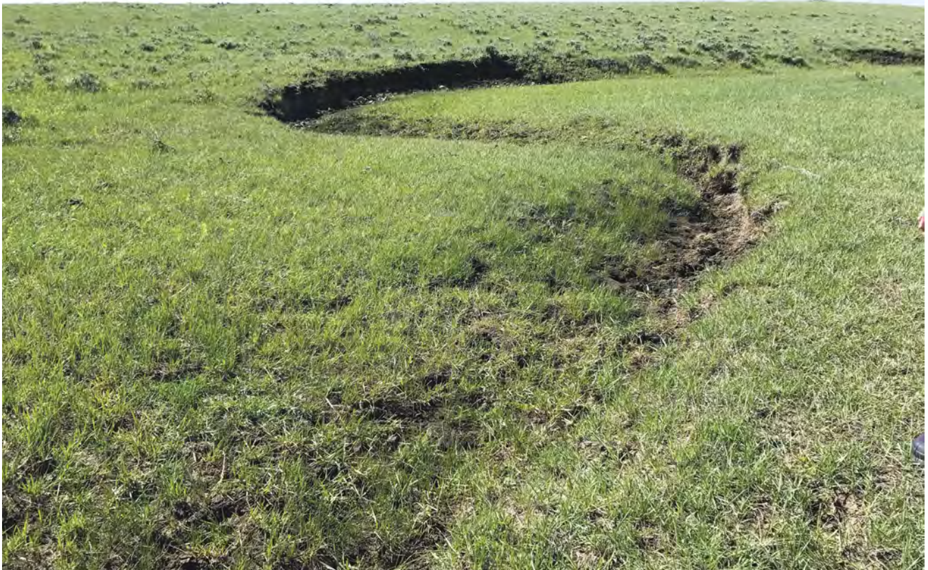
Figure 51: Headwater streams can be particularly vulnerable to overutilization, which results in a loss of vegetative cover. This creates a risk of headcuts and incision in the stream during high-flow events, even if water is only present after rainfall. Photo © Corissa Busse, TNC
