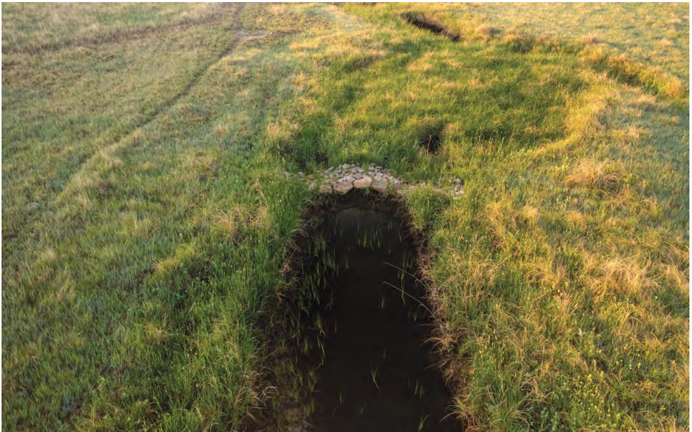
Figure 3. The Zeedyk rock structure shown is trapping sediment behind it, healing a headcut that had formed by filling in with new grass. Photos © Joe Dickie, Generation Photography, Inc.
