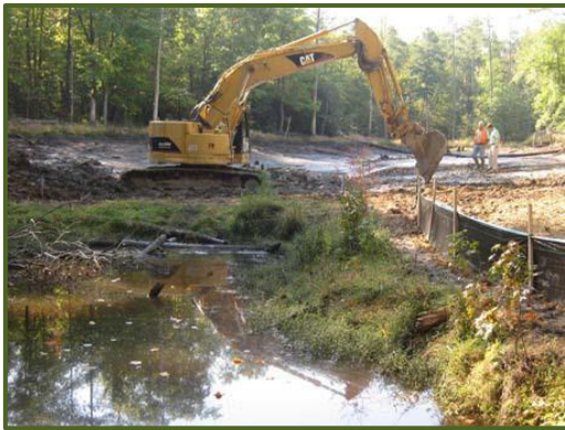
October 2010: Construction begins on the lower dam.
