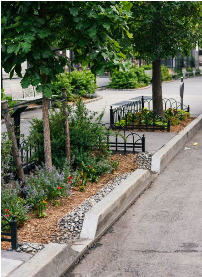
Figure 3.9 Bioswales are a type of green infrastructure used for stormwater mitigation. Source: Kevin Arnold.
